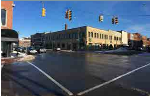
MONROE ST & FRONT ST INTERSECTION
